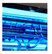
Ultraviolet C (UV-C) technology has been a popular method for preventing the accumulation of airborne pathogens on HVAC equipment for many years now. UV-C bulbs
